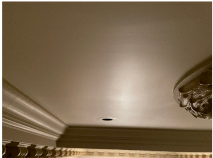
Sample of new surface finish. The forward portion of this picture is the section the fell onto the pews and aisle
