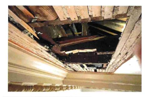
Damaged ceiling joist – cutout of the ceiling showing the joist which was severely notched (lower part of the joist), causing it to crack entirely across (upper part of the joist). Repair to occur next week.
