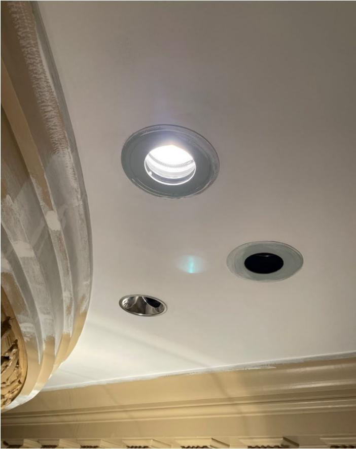
A portion of ceiling next to the dome showing the new skim coat of plaster. Also note the surface repairs on the dome molding in preparation for paint. Most of the spackling for paint prep on the molding and coffers has been completed.
