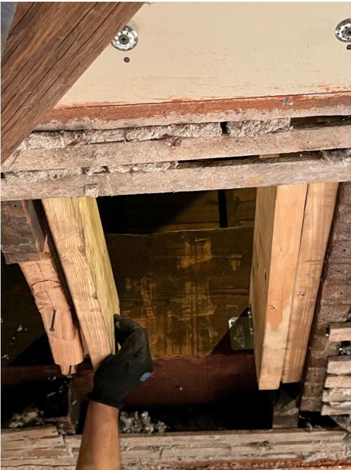
New joists being installed at the location where the original joist had cracked through. The ceiling needed to be jacked into place to line up with the beam because the ceiling area had significantly sagged
