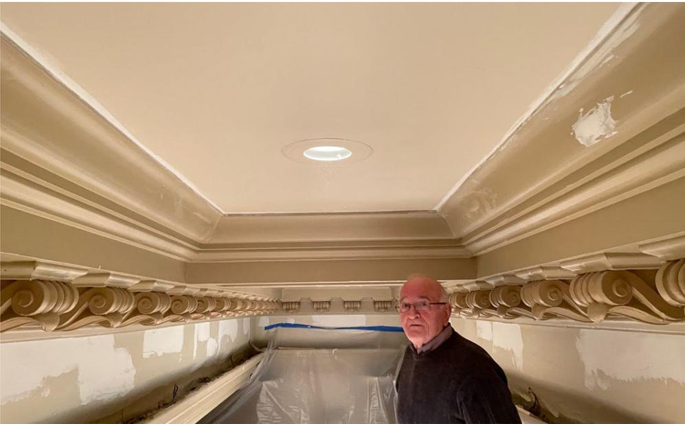
Portion of new ceiling that has been skim coated and test painted (including inspection by maintenance committee member extraordinaire, Van Paras). Petrinis Painting matched the paint color by removing chips of the 4 colors in the ceiling and tested the match and application prior to the paint crews arriving next week
