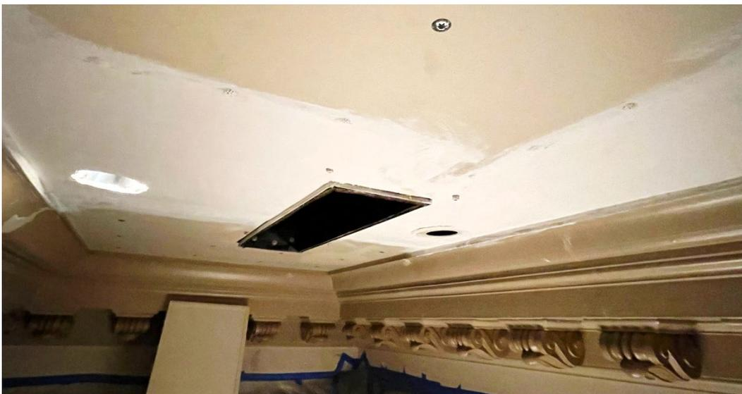
New plaster in two different coffers. The black rectangle is the air conditioning duct with the cover removed.
