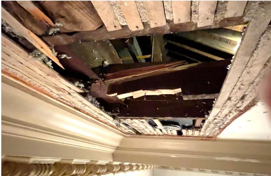
Damaged ceiling joist – cutout of the ceiling showing the joist which was severely notched (lower part of the joist), causing it to crack entirely across (upper part of the joist). Repair to occur next week.
