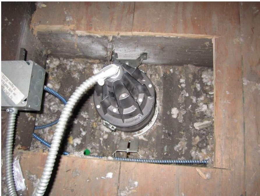
Figure 5. Light adjacent to failure area with no evidence of moisture.
