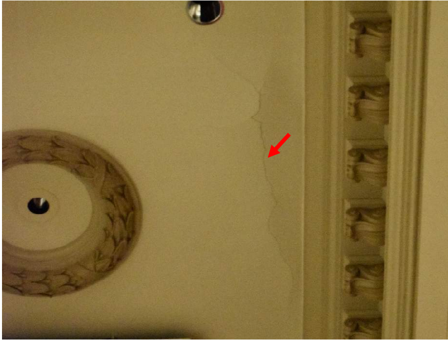
Figure 12. Cracked and bowed plaster at the north aisle.
