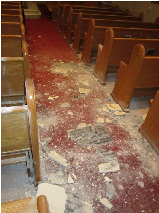
Figure 2. Fallen plaster at the south aisle.
