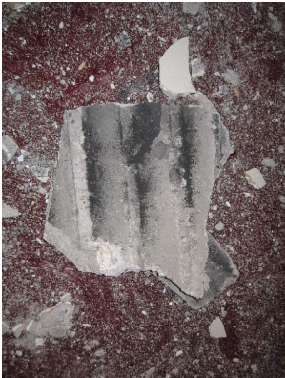
Figure 9. Fallen plaster with evidence of top-side soiling (darker areas), indicating previous debonding between the plaster and the wood lath.
