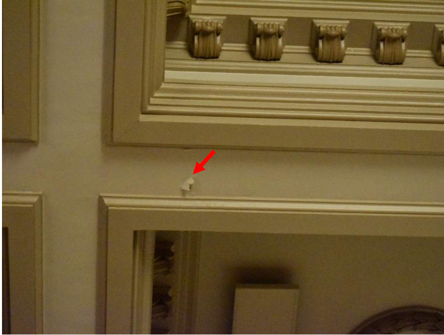
Figure 14. Peeled plaster coating at beam. Multiple similar conditions were observed on the sanctuary ceiling.
