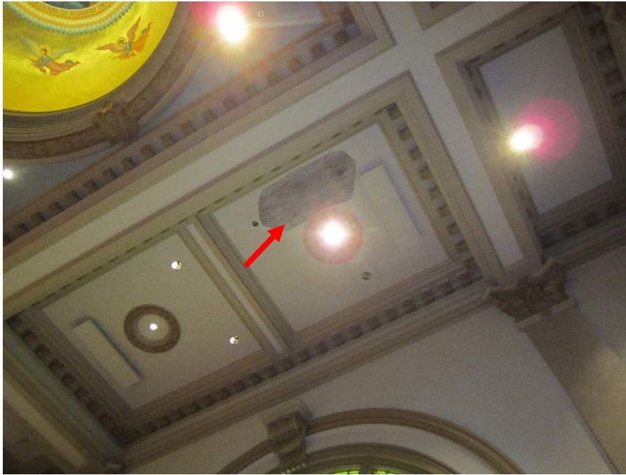
Figure 1. Area of plaster collapse; viewed looking toward south wall of sanctuary.
