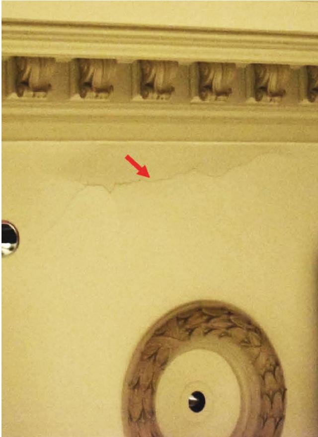
We did finally receive the report from WJE. The contents were in-line with what they have been discussing with us along the way. One good picture included in their report is a second large area where the plaster has cracked and bowed down away from the lath.
