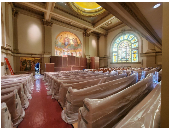
Pews wrapped. Scaffolding will stand between pews.
