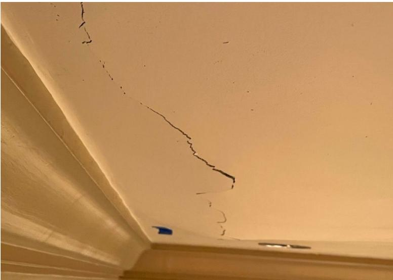
This is a close-up of the other large crack that was visible from the ground. The crack is over 6 feet long and the plaster is clearly bowed downward.
