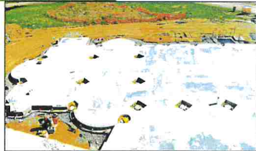
Chapel concrete slab poured
